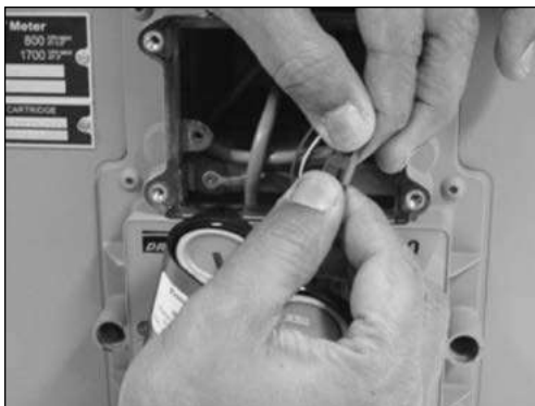
Figure 9.30 - Disconnect the wiring
