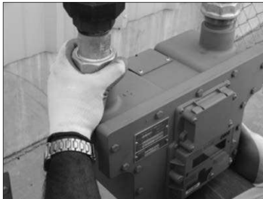
Figure 7.2 - Connect meter ferrule into swivel nut on the gas supply side
