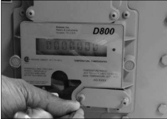
Figure 9.1 - Remove two button head screws
