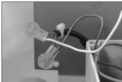
Figure 7.20 - Pulse Output 2 wired to the ERT with a cable tie located near the end of the shrink tubing
