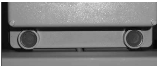
Figure 7.27 - Red tamper seals installed
