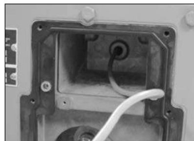
Figure 9.16 - Run cable through back of meter
